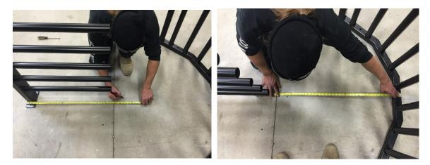
10. Using a square, on the 33" mark make a line perpindicular to your center line, place the rotor bearing mounting plate corners and mark and drill the 3/8 anchor holes.
