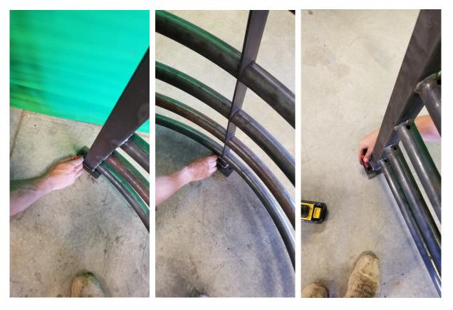
8.DRILL AND ANCHOR ALL 8 CAGE AND COMB MOUNTING HOLES. TIGHTEN ALL ANCHORS AND HEADER BOLTS.
