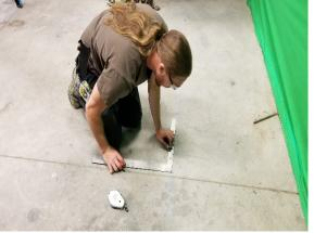
10. USING A SQUARE, ON THE 33" MARK MAKE A LINE PERPENDICULAR TO YOUR CENTER LINE, PLACE THE ROTOR BEARING MOUNTING PLATE CORNERS AND MARK AND DRILL THE 1/2 ANCHOR HOLE.
