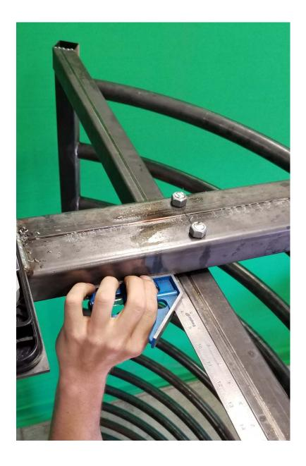
7. ONCE TURNSTILE IS IN DESIRED LOCATION AND SQUARE AND PLUMB, MARK THE HOLES FOR ANCHORING IN COMB AND CAGE.
